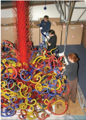
Glass team installing Fireworks of Glass on steel armature
